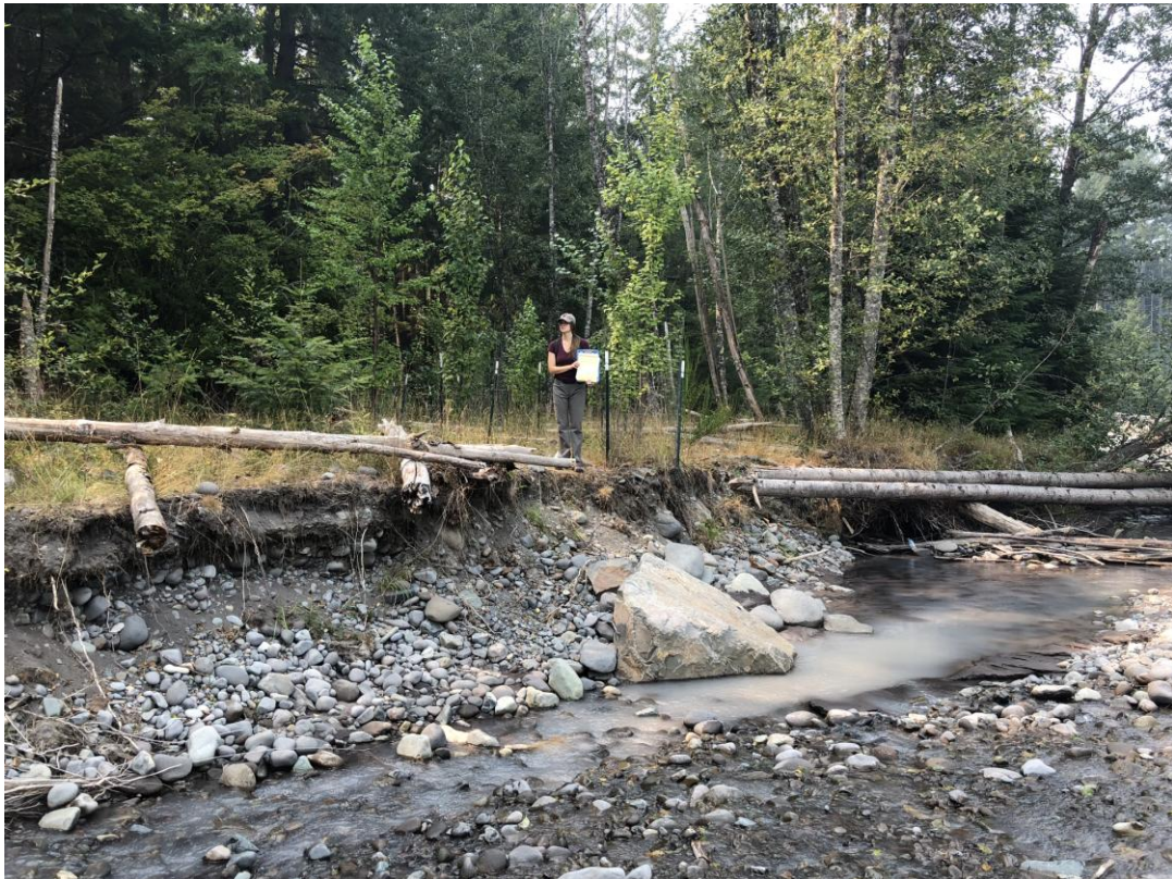
Vane 11 remains one of the highest eroding banks. Here note the large boulders that comprise the now-exposed vane. Toe erosion is contributing to large overhanging banks.
