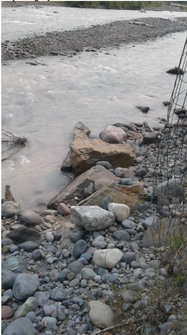
Vane 4 has a section of the vane exposed (larger angular rocks).
