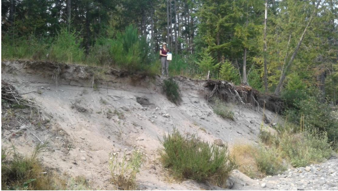
Vane 6 establishing vegetation at toe since flow has been less frequent at the toe over the past few years.
