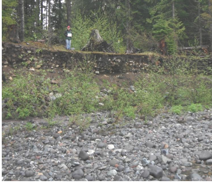
Vane 5 area is setback from the deepest part of the channel and although experiencing some chronic erosion at higher flows, over the last couple of years vegetation has established at the toe.
