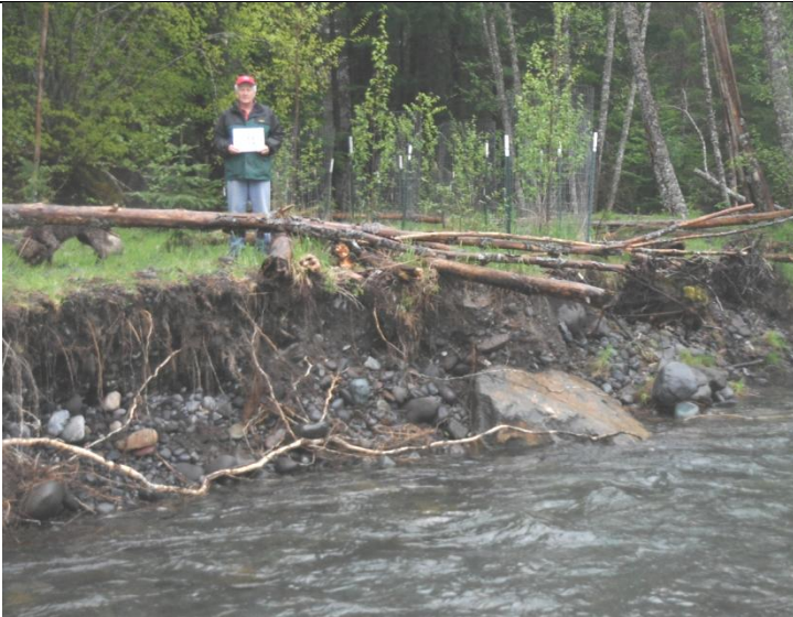
Vane 11 is exposed to flowing water at all river levels at this time and actively eroding. Portions of the buried vane are exposed as evidenced by the large boulder in the foreground.
