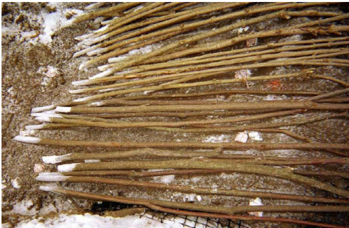
Live cuttings are dipped in rooting hormone before installation
