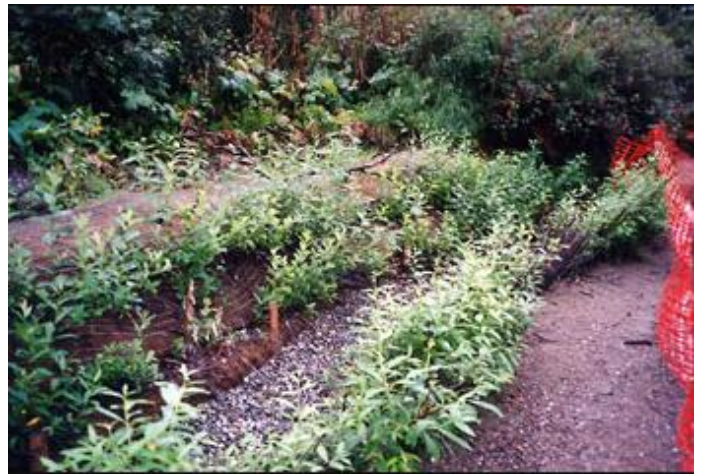
Combining bundles with live stakes is an effective toe erosion application and helps to trap sediment
