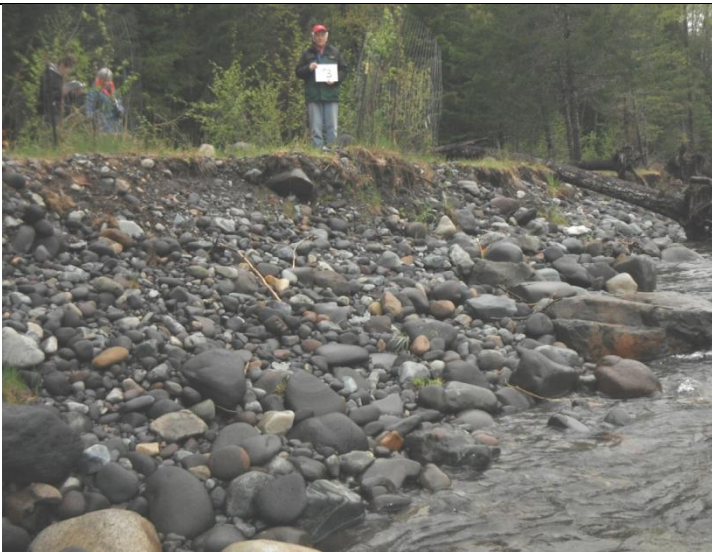
Vane 3 area is experiencing active toe erosion and slight exposure of the buried vane.
