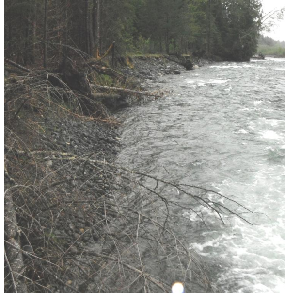
Vane 2 (background) and Vane 3 (foreground) areas have active toe erosion at normal flows.
