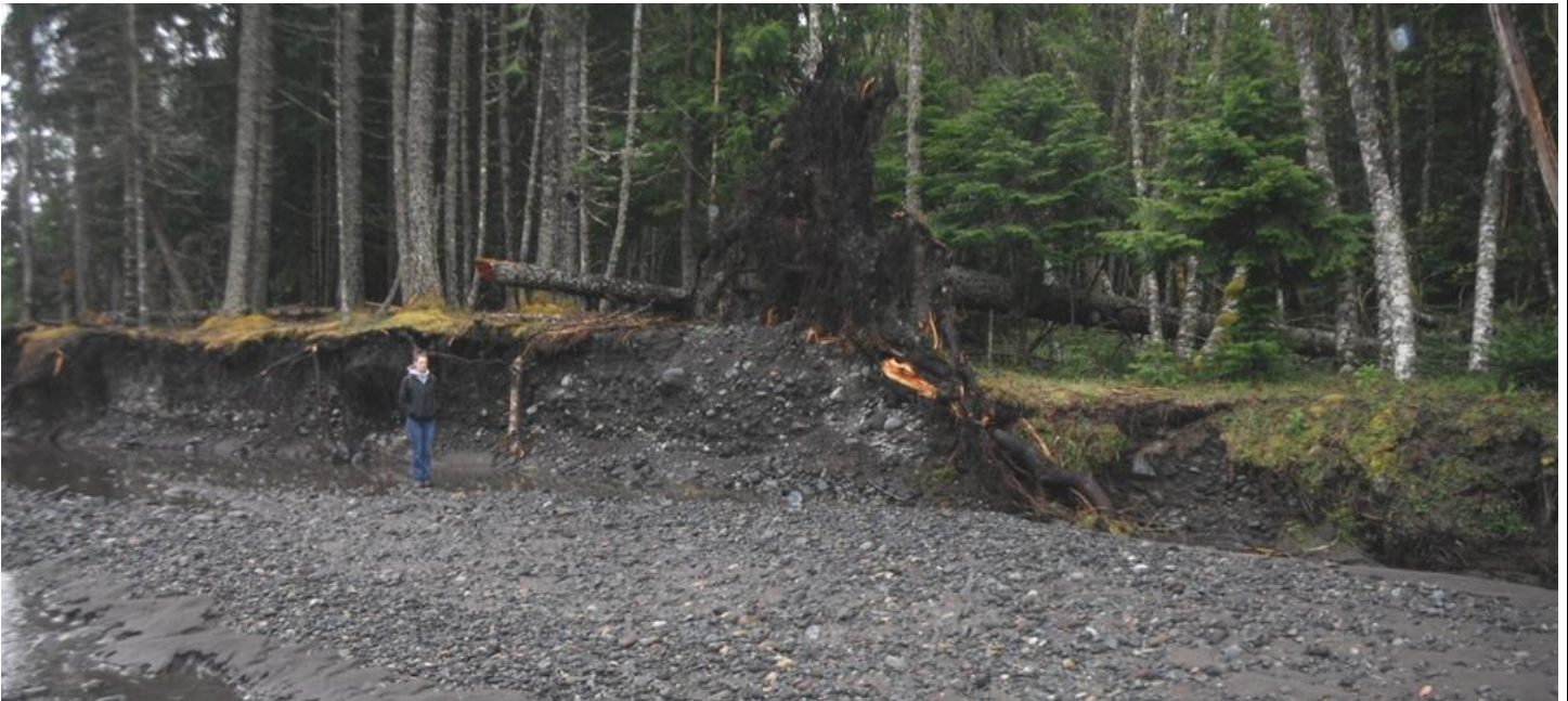
The area between vanes 12 and 13 is exposed to flowing water at flood levels and is highly undercutting. Newly fallen trees, large trees on undercut banks, loosely consolidated bank material and direction of flows during flood events make this area a candidate for severe erosion in coming years.
