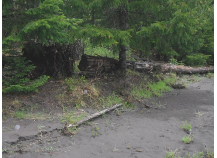
Vane 10 area has been largely unaffected through the evaluation. Fine sediment deposition occurs during flood stage due to downstream structure causing backwater. This area is a candidate for vegetation establishment before the downstream structures break apart and the backwatering effect is lost.
