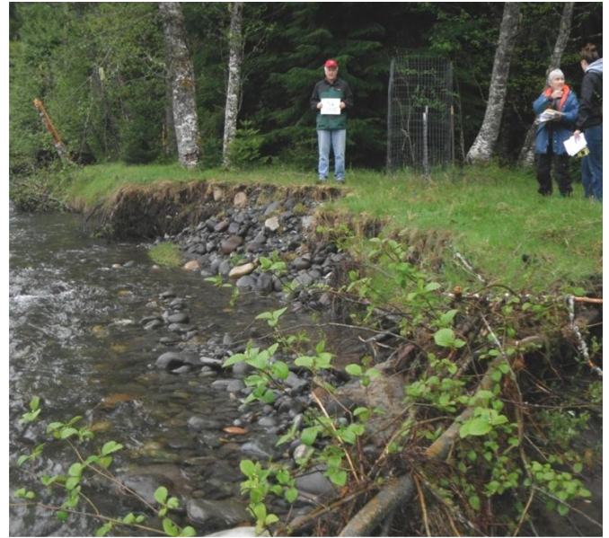
Vane 14 area is experiencing active toe erosion at normal flows. Loss of bank upstream is contributing to increased exposure and this area can be expected to see increased erosion rates in coming years.
